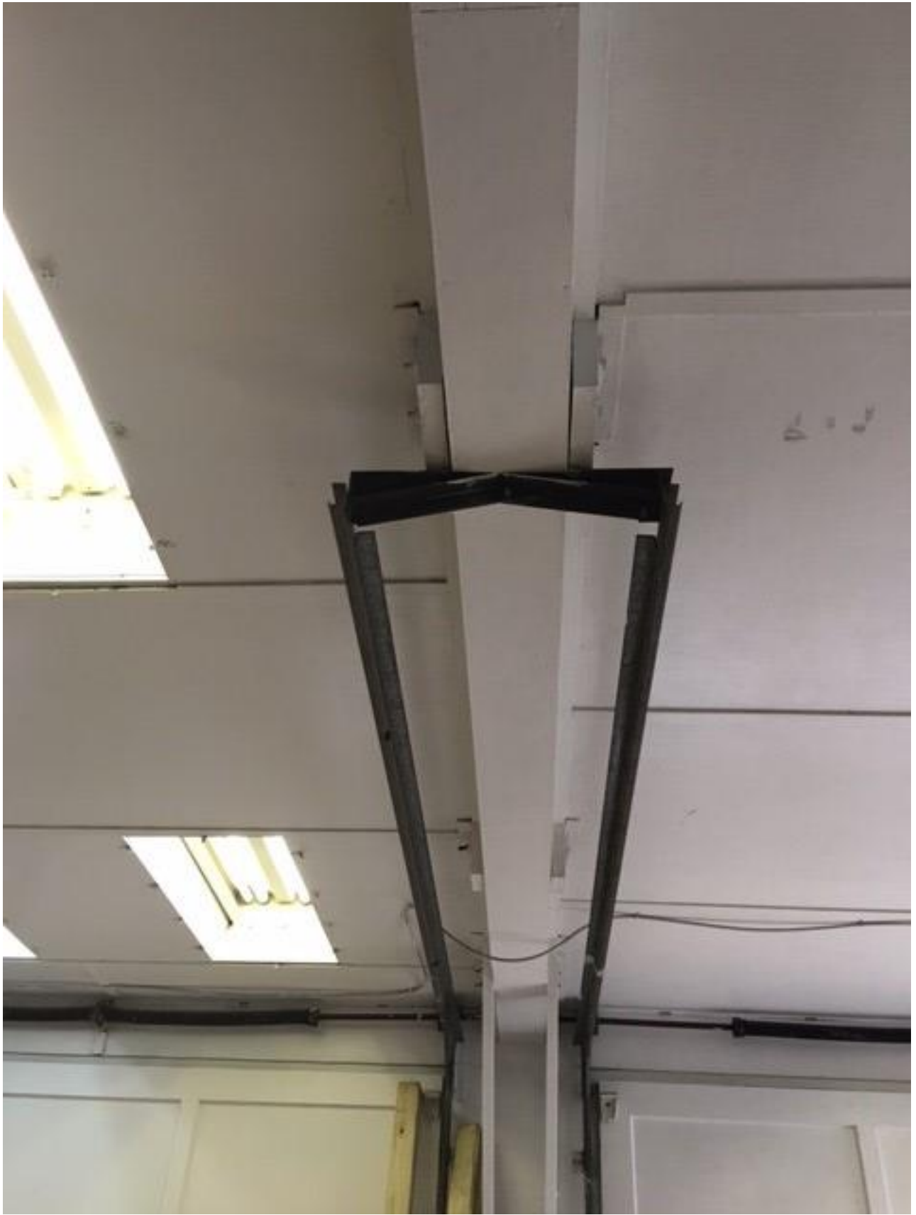
INTERIOR OVERHEAD TRACK
