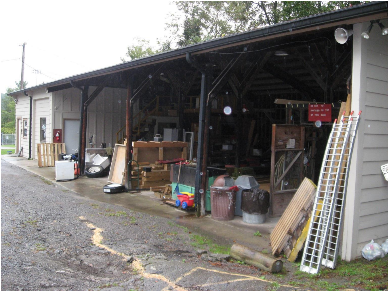
SIX BAY POLE BUILDING
